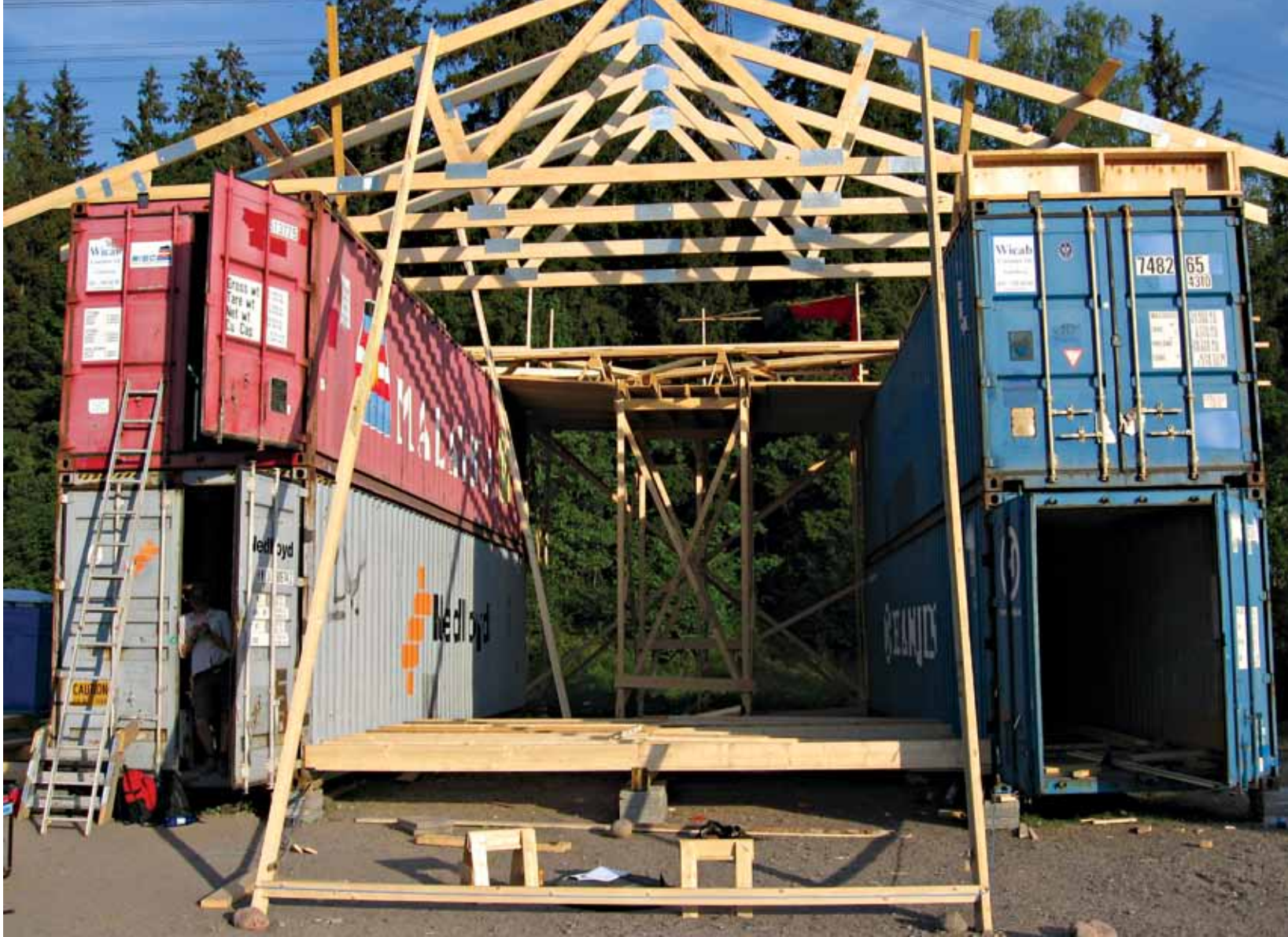
Using traditional methods, we built and raised the roof trusses by hand.
