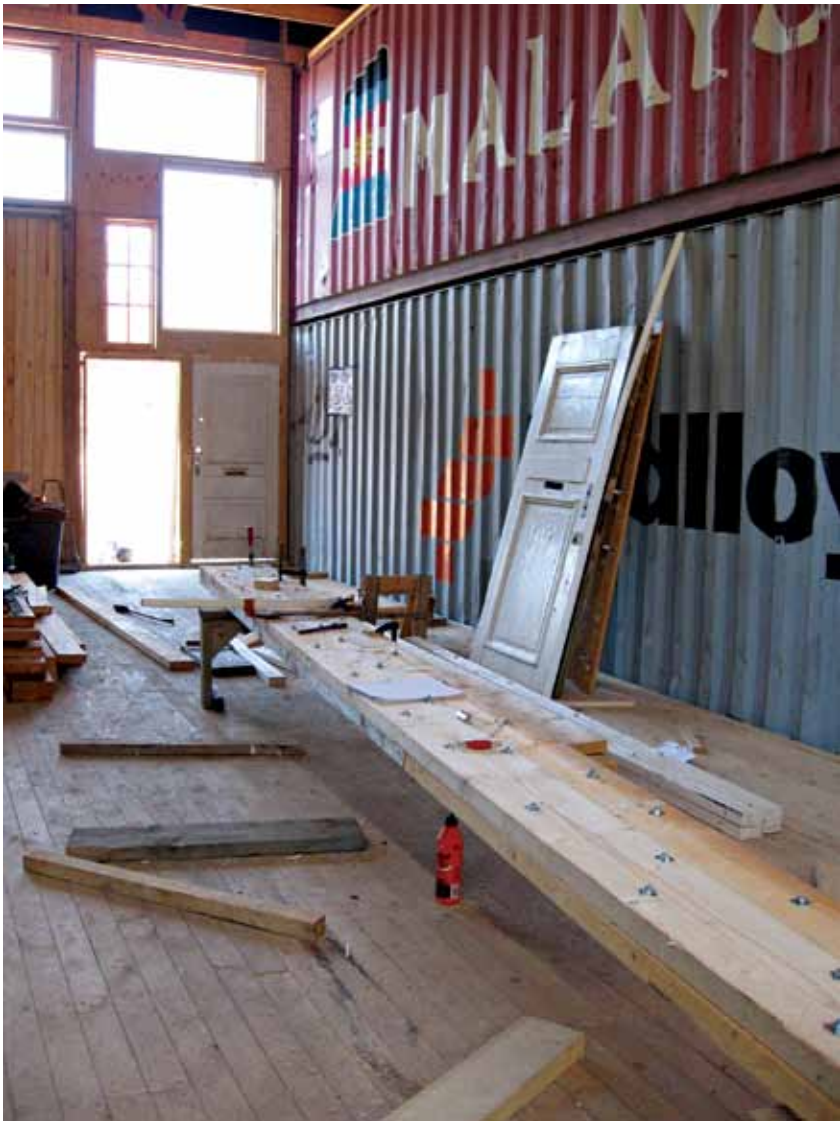
Instead of buying expensive glulam beams, we made our own out of plywood, bolts, and good old PVA carpenter's glue.
